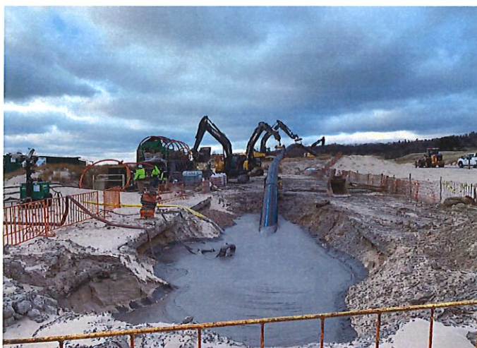
Pipe entering north pit during pullback
